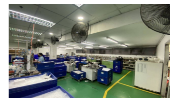
Replaced air conditioners with air-cooled chillers Janome Thailand, Co., Ltd.
